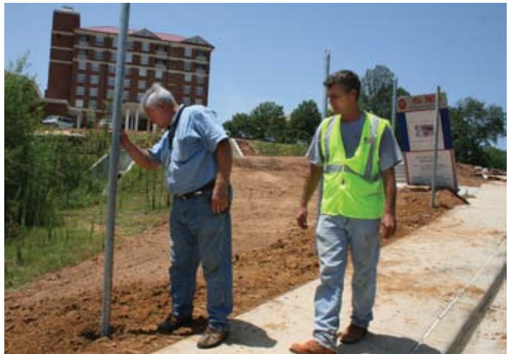
Morris Horn, University of Mississippi (left) and Freddie Gurley, UtiliQuest, check the progress on the 7000’ security fence on the Ole Miss campus.
