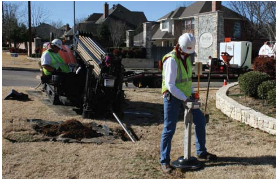
(Top) Klaasmeyer subcontractor, Wyonna Burckhard of Burckhard Contractors locates the boring head as Jason Burchard operates the directional drilling rig.
