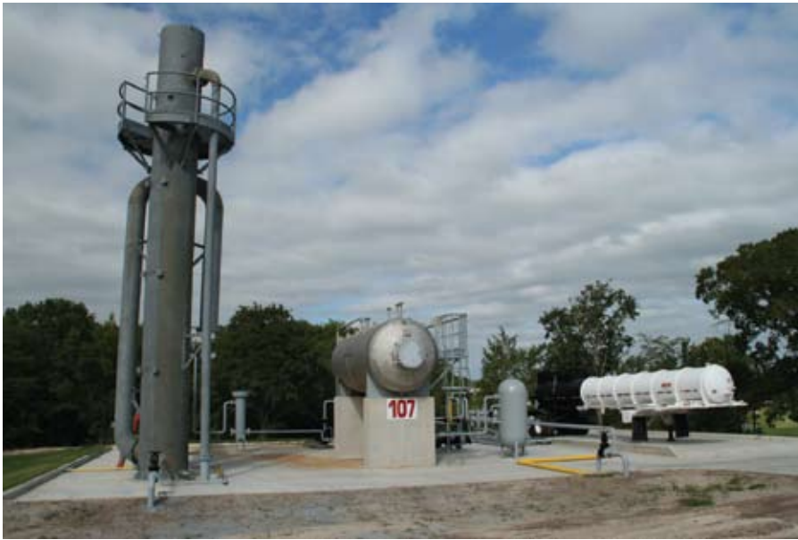
(Top) The recently completed TEEEX pipeline training prop.
